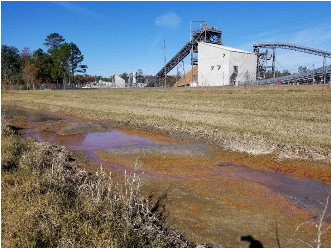
Figure 9. Sediment Accumulation in the Northern Drainage Ditch
