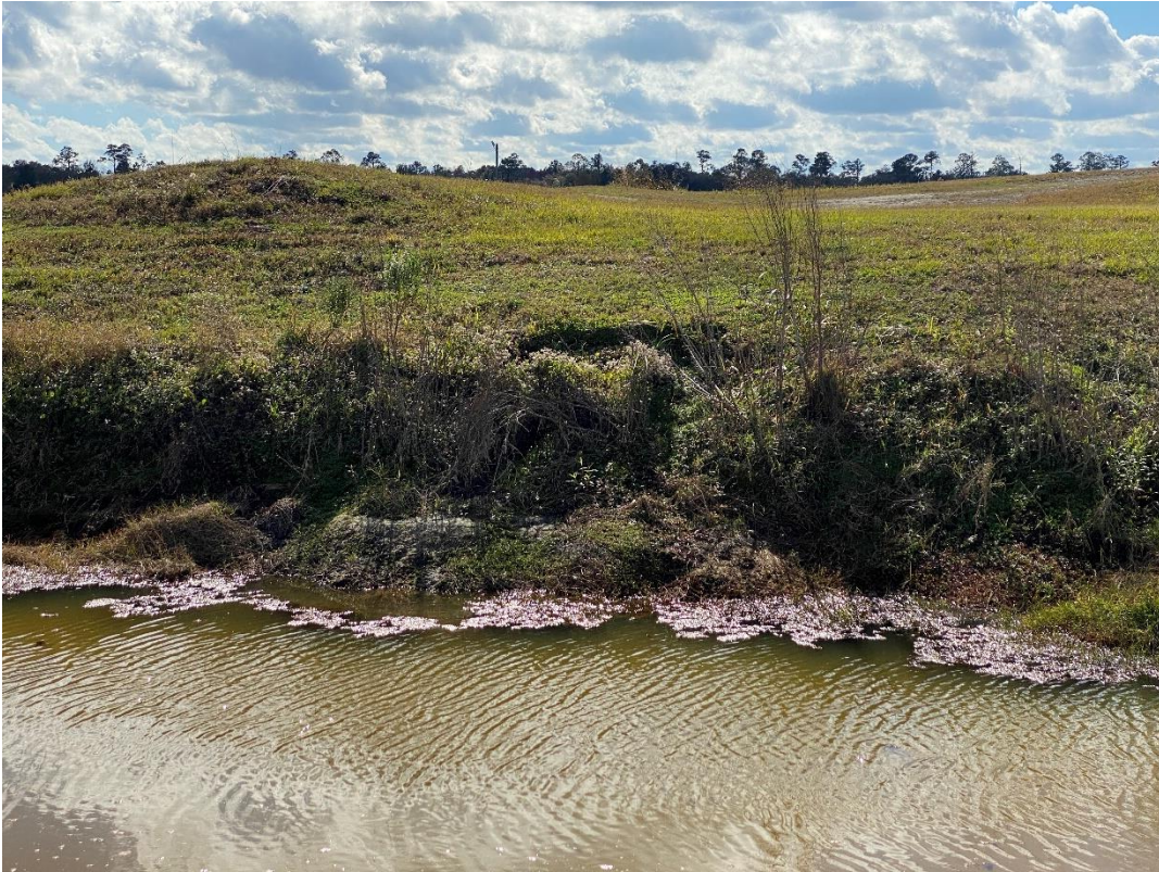
Figure 6. Erosion near the Southeast Corner of North Drainage Ditch
