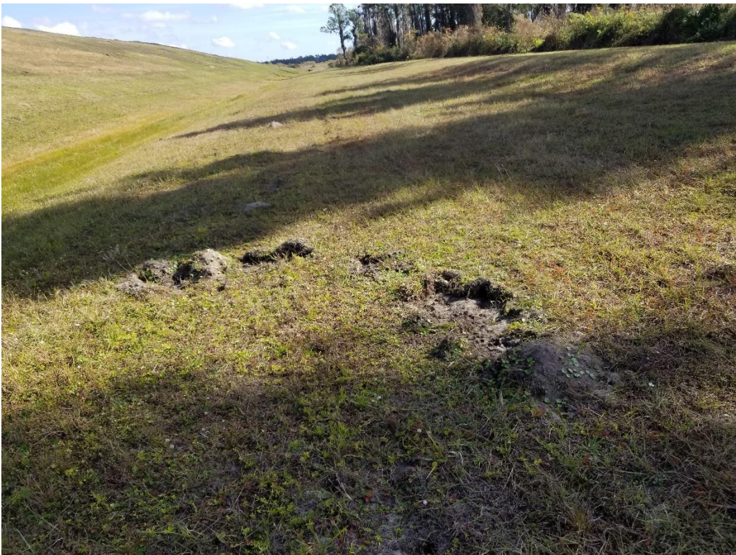
Figure 11. Unvegetated Areas in Stormwater Channel on the South and West Side of the Landfill
