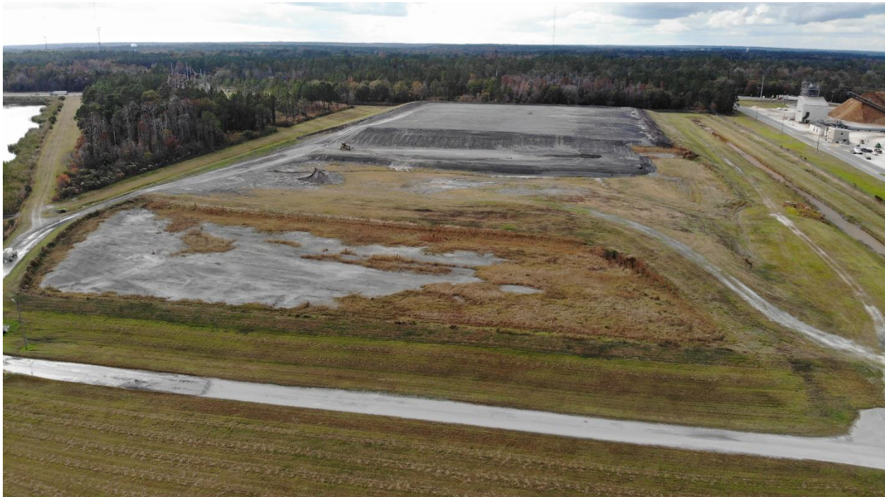
Figure 2. Aerial Image of CCR Landfill Facing West
