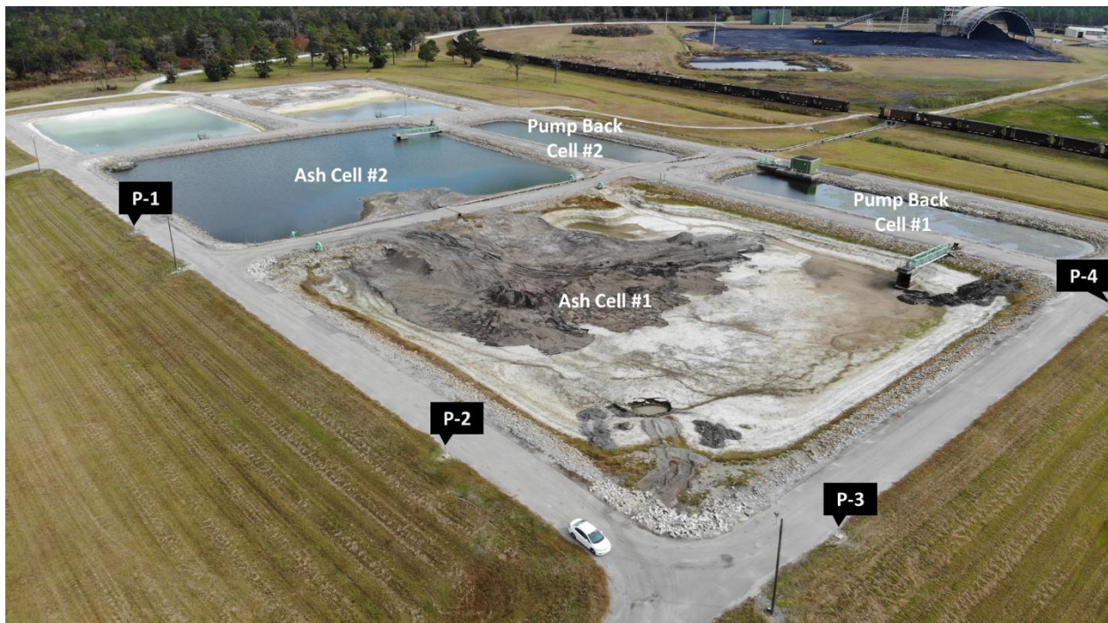
Figure 1. Layout of the CCR Surface Impoundment System, Adjacent Pump Back Cells, and Piezometers
